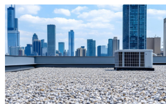
ROOFTOP INTRUDER DETECTION
