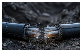
NETWORK DAMAGE, CUTS AND THEFT
